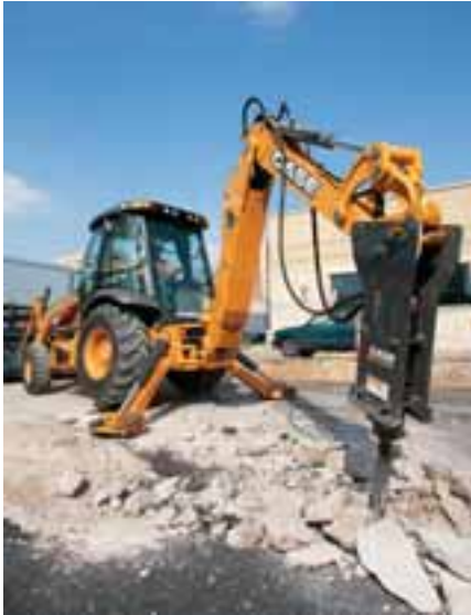
Optimized hose routing for demolition work
